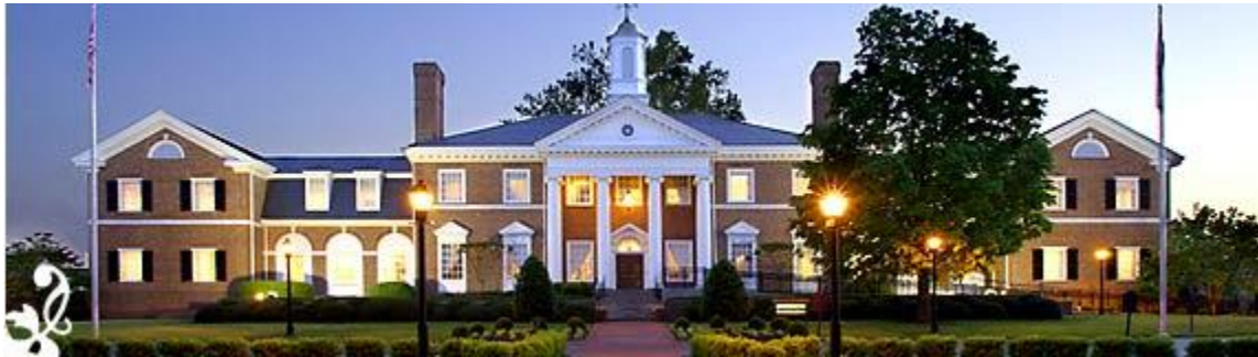
Virginia Crossings Resort Hotel
